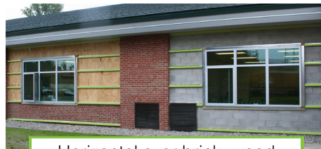
Horizontal over brick, wood & CMU with spray foam
