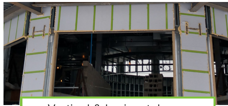
Vertical & horizontal over metal stud with polyiso
