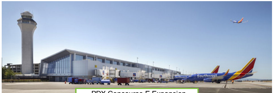
PDX Concourse E Expansion Portland, OR
